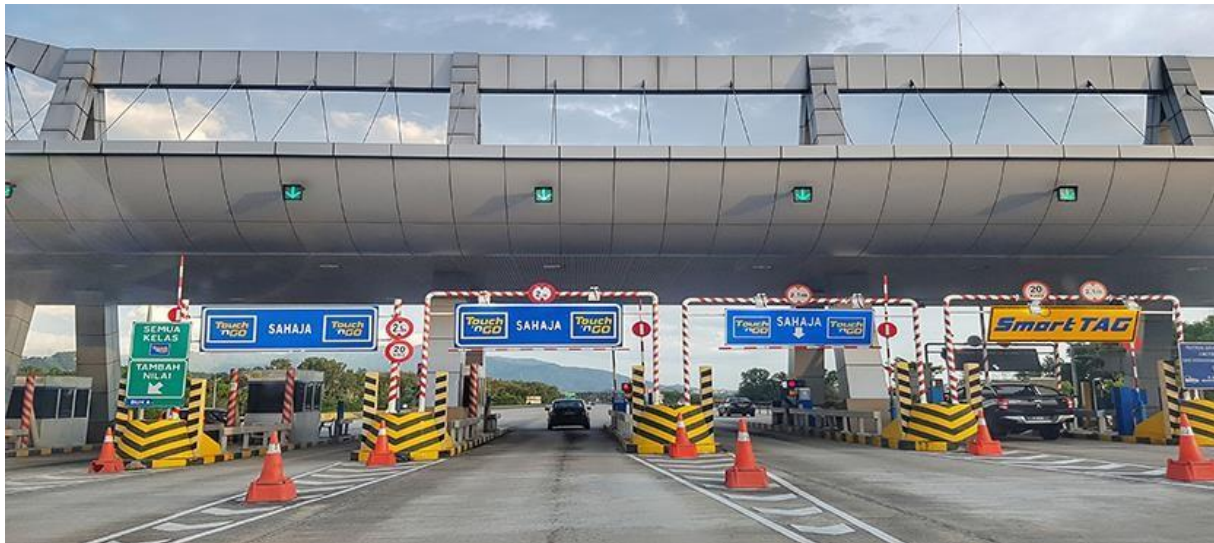
Figure 4.4.14: Highway toll gate in Malaysia using a universal prepaid chip card „Touch ‘n’ Go“ ( https://www.comparehero.my/blog/use-touch-n-go-card )
