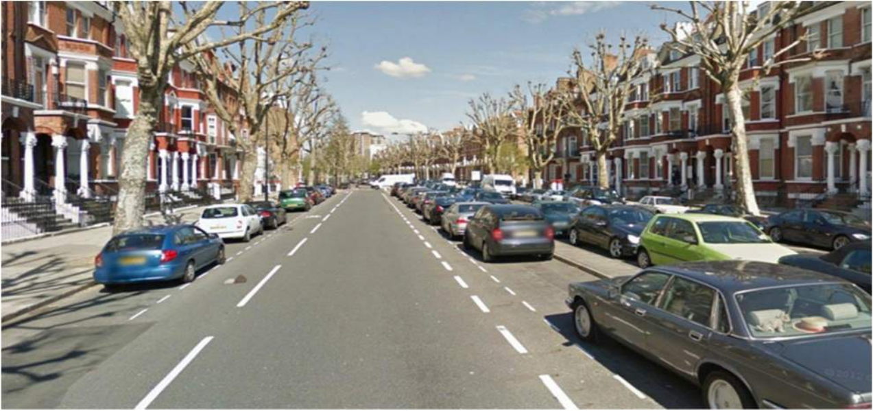
Photo 3.7 – Example of thermoplastic paint used to demarcate bays on a tarmac surface
