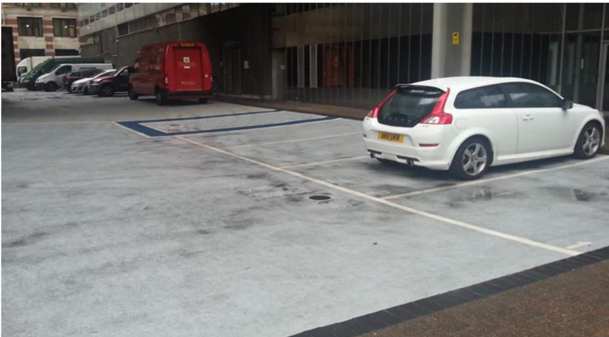
Photo 3.8 Example of thermoplastic paint used to demarcate bays on a concrete surface
