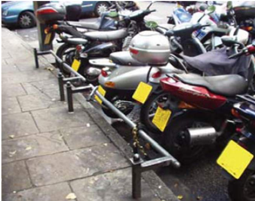
Photo 3.2 – Example of a stand-alone motorcycle anchor rail
