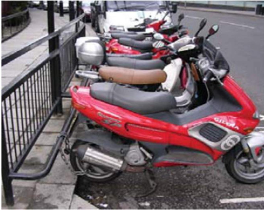
Photo 3.3 – Example of motorcycle parking with continuous rail integrated with pedestrian guard railing
