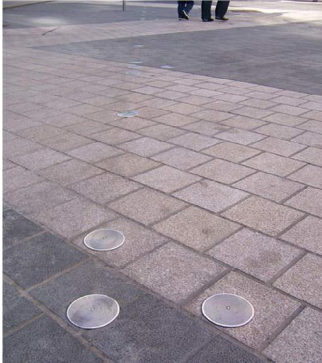
Photo 3.9 – Example of metallic studs used to demarcate bays
