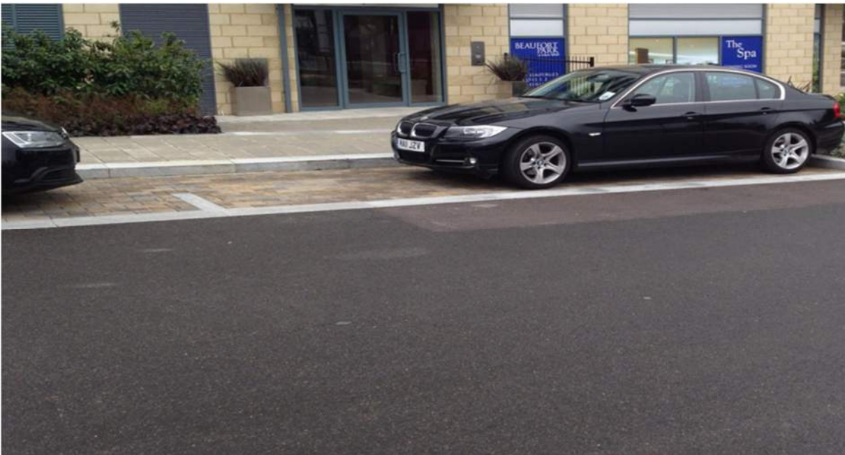
Photo 3.6 – Example of block pavers used to demarcate bays
