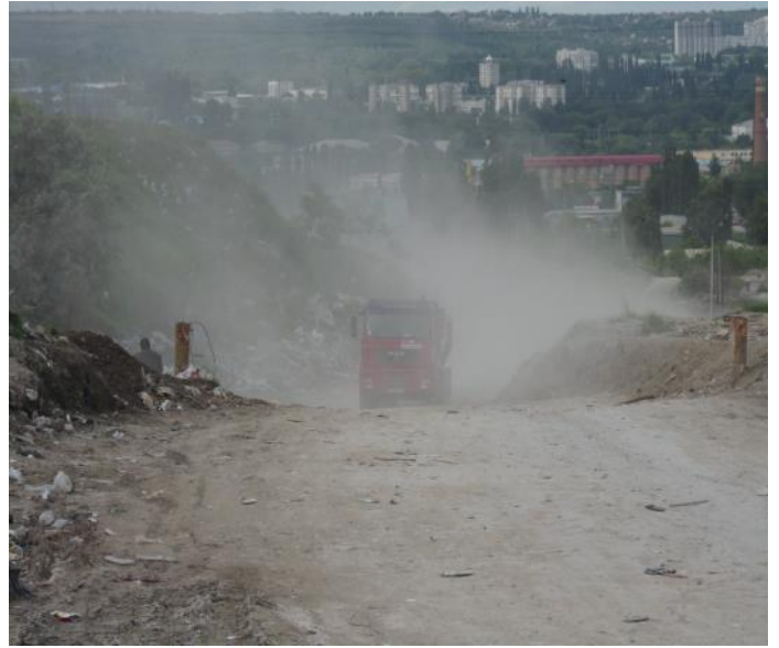
Poor road surface within the site, significant dust re-suspension
