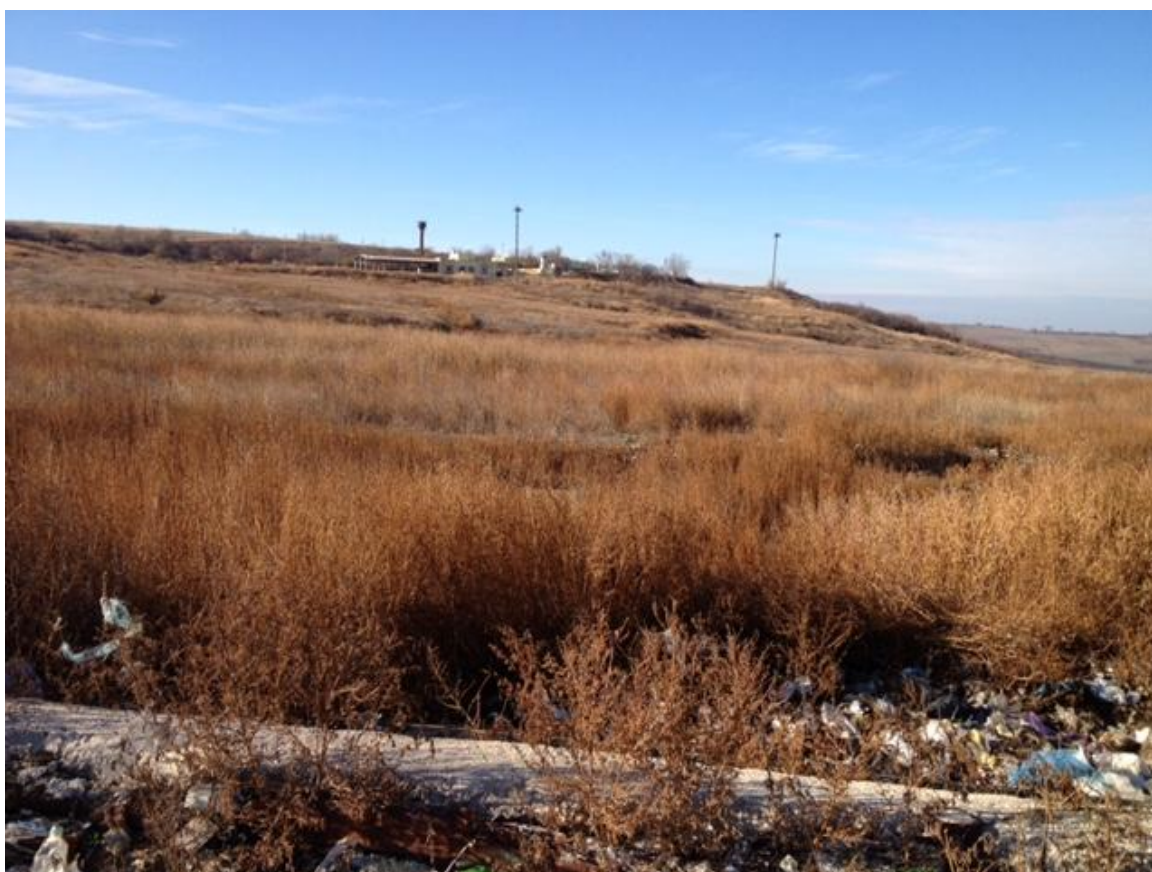
Figure 11-1 View looking west across Tintareni landfill site towards the biogas plant
